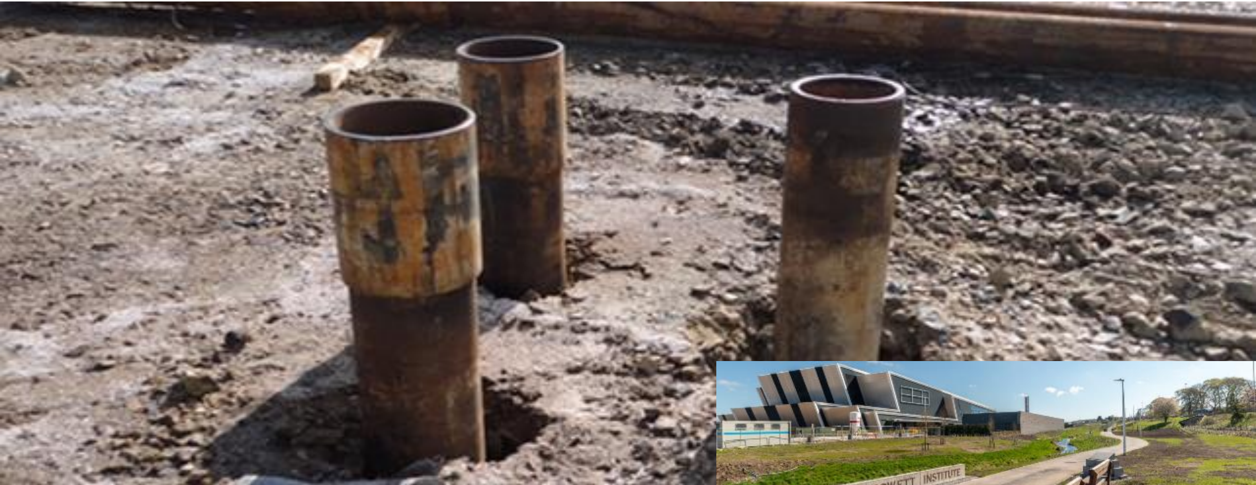
O&G pipes for piling
