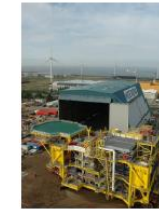
Fabrication Yard Vlissingen
