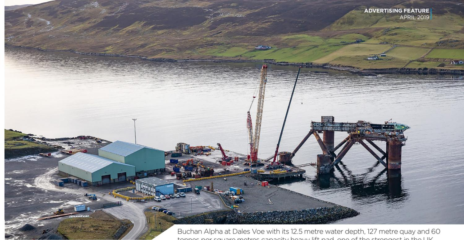
Buchan Alpha at Dales Voe with its 12.5 metre water depth, 127 metre quay and 60 tonnes per square metres capacity heavy lift pad, one of the strongest in the UK.
